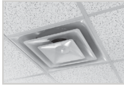
Supply diffuser(s) that connect to fan assembly
